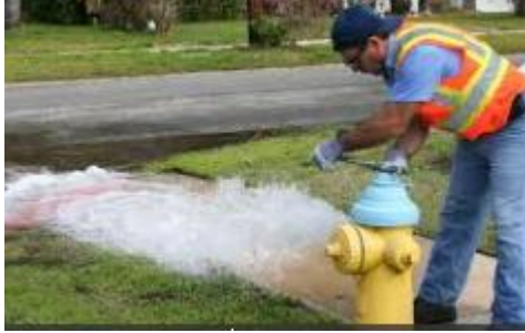
Water Company worker checking a hydrant.
