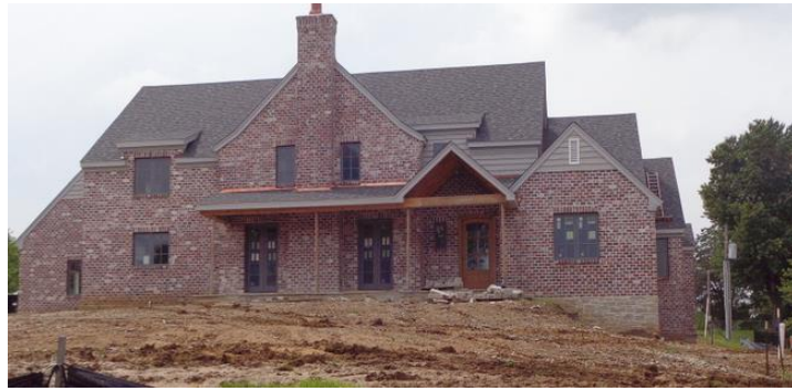
New House under construction
