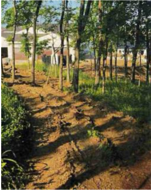
Heavy Equipment Damage in green space Protected Tree damage
