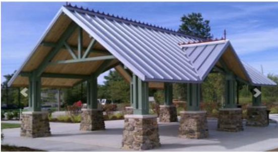
Alternate 1: Standing Seam Metal Roof (above)
