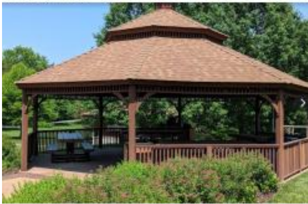
Pavilion before fire, unfortunately it appears
