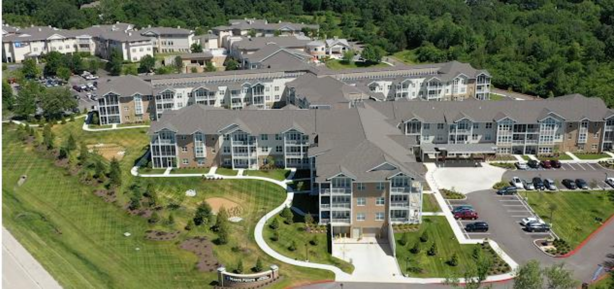
Current Mason Pointe facility
