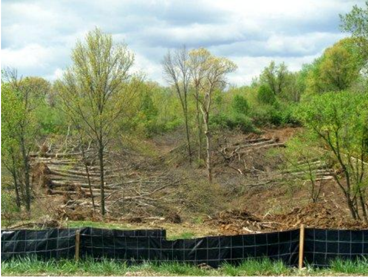
View of the project from April 20, 2015.
