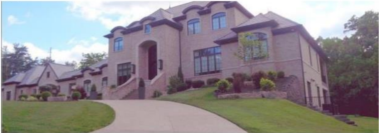
601 Greenwich Green on the side rear lot of the former house that faced Clayton Rd.
