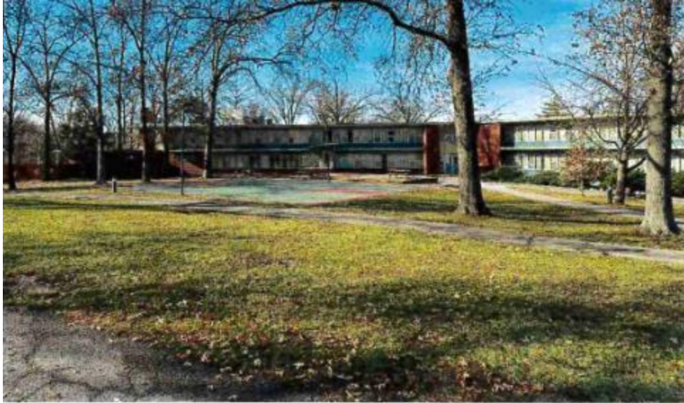
Photo #10 – Existing Dorm Building (To be demolished) – Looking northwest
